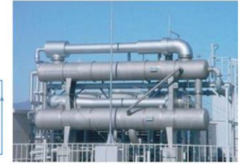
Fig. 5: 2-stage steam jet cooling plant of compact design, cooling 44 m 3 /hr of water from 30 to 10 °C.
