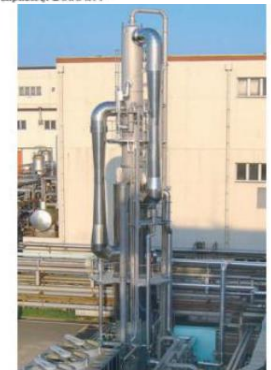
Fig. 7: 2-stage steam jet cooling plant of column design, cooling 250 m 3 /hr of water from 10 to 5 °C.
