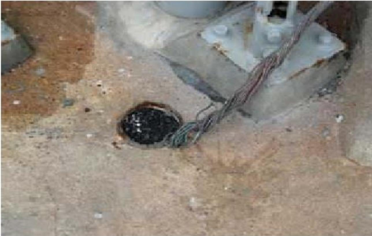
Defective bonding strap shows poor maintenance.
